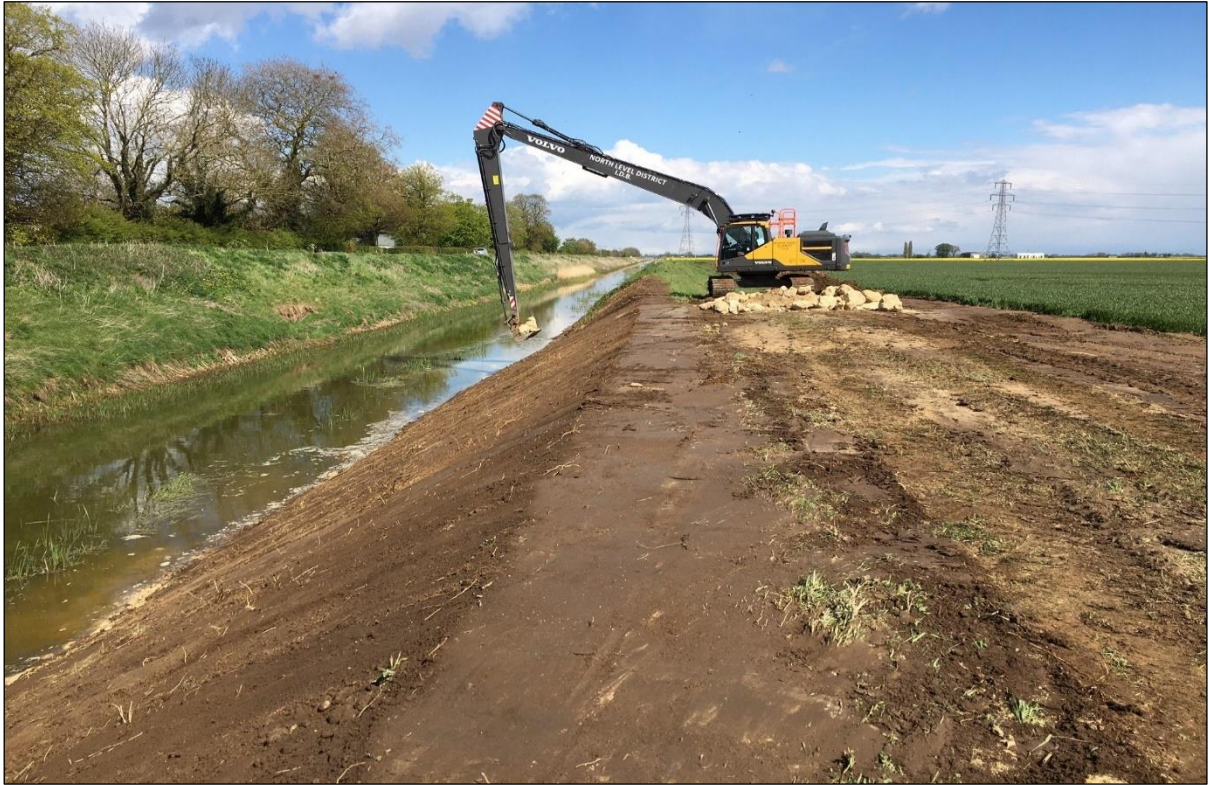
New South Eau bank repair
