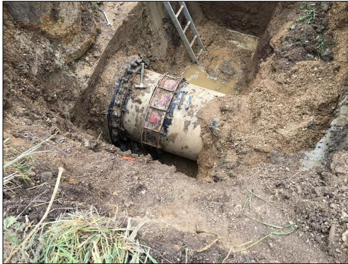
Split visible within the fibreglass discharge pipe
